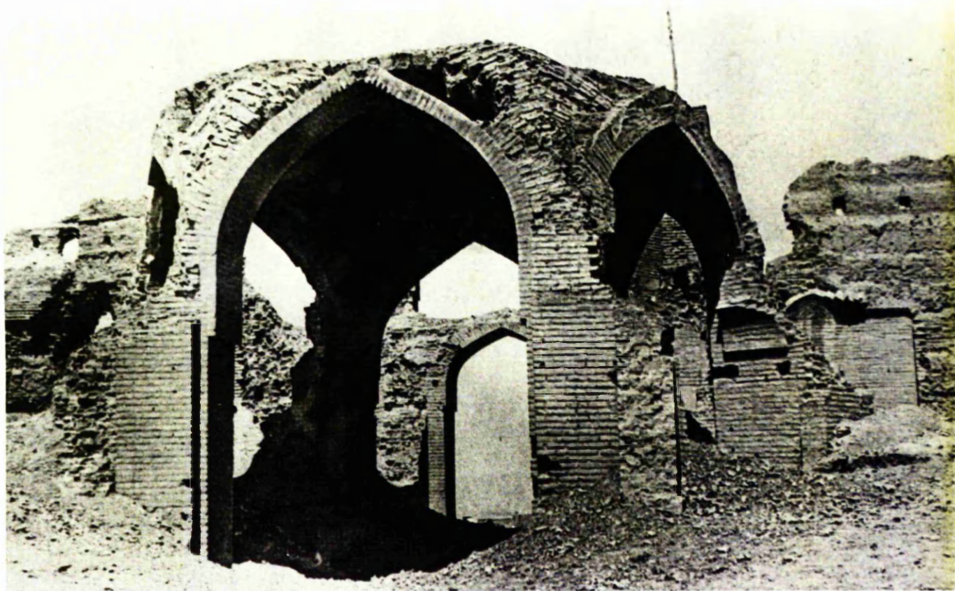
Pl.9. Caravansarai Sin. Vault at a corridor crossing.
