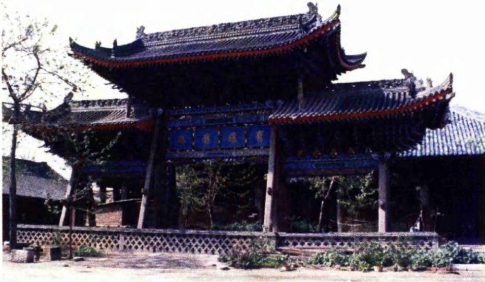
Fig. 3.1 The front temple of the old Chenghuang miao Daoist Monastery built in 1384 and destroyed during the Cultural Revolution. The site is now an open-air market.
