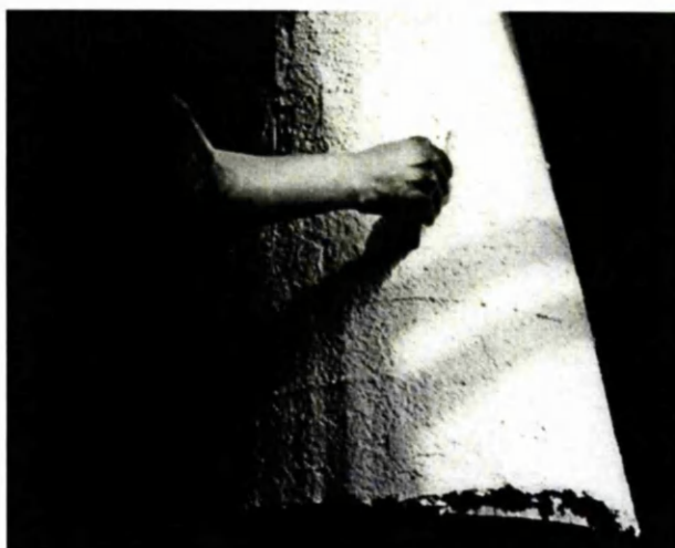
On the third frame Ikram applied a smooth plaster finish and some painted clay shapes in the apex.
