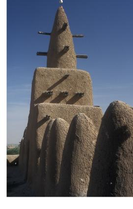
with quantities of chopped straw, dry rice husks, or cow manure, and less commonly with tiny pebbles, ash, earth from termite mounds, powdered baobab fruit, or *karité* (shea-nut) butter. Left to ferment, the additives improve cohesion, durability, and water resistance.
